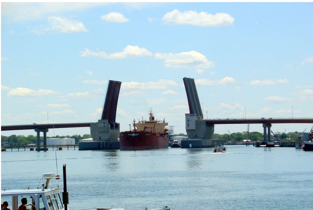
Figure 15. Photograph of Casco Bay Bridge. Digitized features include the two main columns supporting the drawbridge and the cylindrical columns to the front and back of the main columns.
