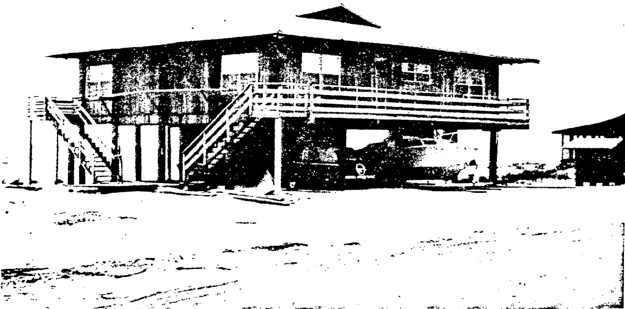
Figure 17. Pole house with integral pole - rigid frame construction.
