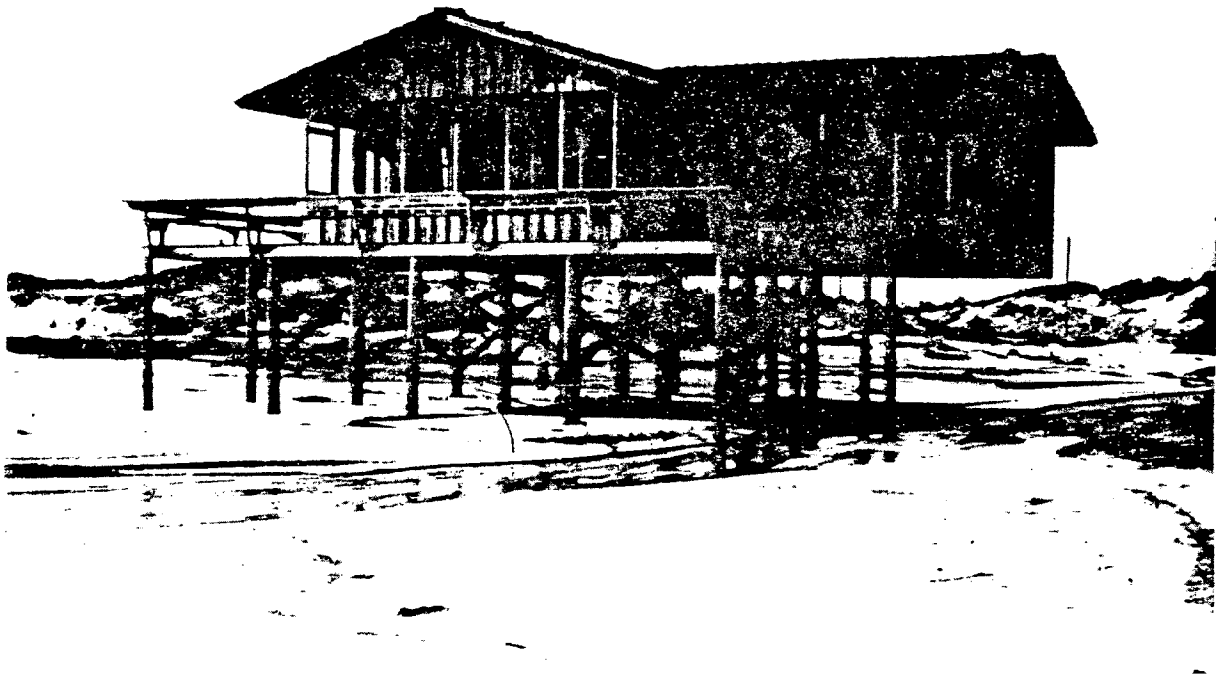
Figure 16. Pole house which survived Hurricane Eloise.
