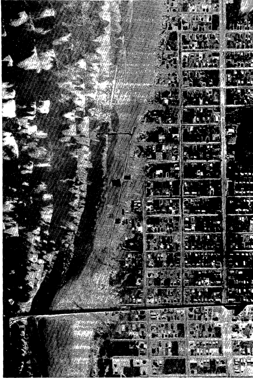
FIGURE 8. 23rd to 38th Streets showing 1962 storm damage in the longshore drift nodal zone. In the absence of street-end dune protection this pattern of overwash will be repeated. The present dune line is still narrow and easily subject to breaching.
