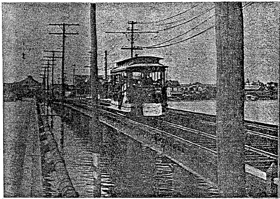
Deal Lake Bridge, 1915
