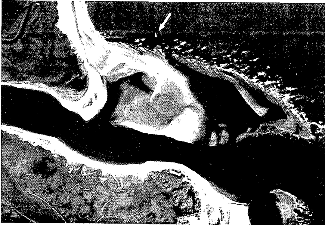
Figure 25. Morris Island light. The lighthouse was located on the beach at the south end of Morris Island in 1939. Over 1600 feet of erosion has occurred since that date. This erosion is in part related to the construction of jetties at Charleston Harbor to the north, as well as its proximity to a tidal inlet. Photo taken January 7, 1975.
