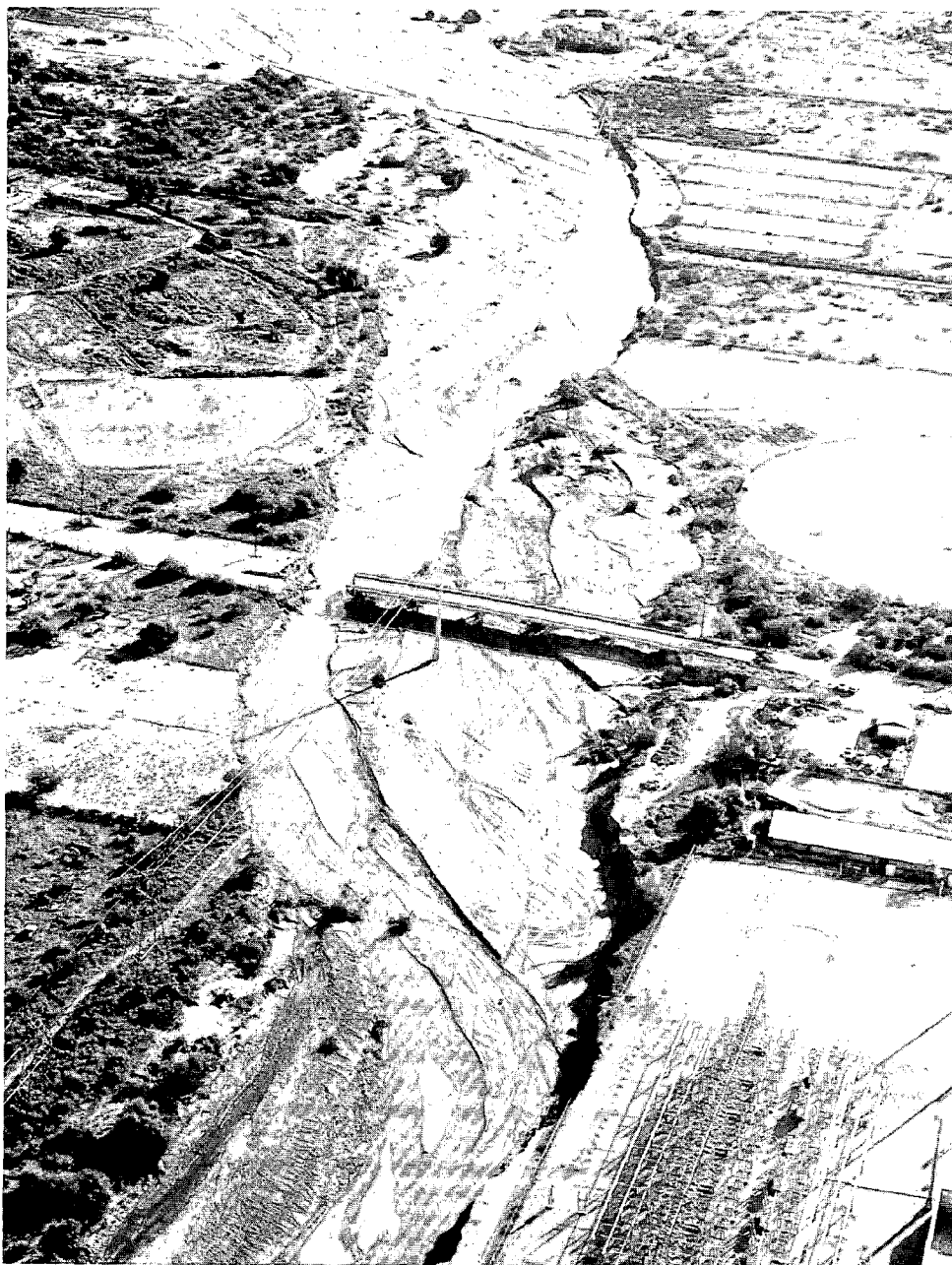
FIGURE 27 The Dodge Road bridge over the Rillito on October 9, 1983. Damage to the north (left) abutment was caused by meander migration. Note the prominent cutbank on the north side and corresponding point bar on the south (right) side of the stream. The meander bend immediately downstream (bottom right) is threatening an electric utility station. The anomalously wide section of channel at the top center was the site of a preflood channel sand-mining operation. Photograph by Peter Kresan.
