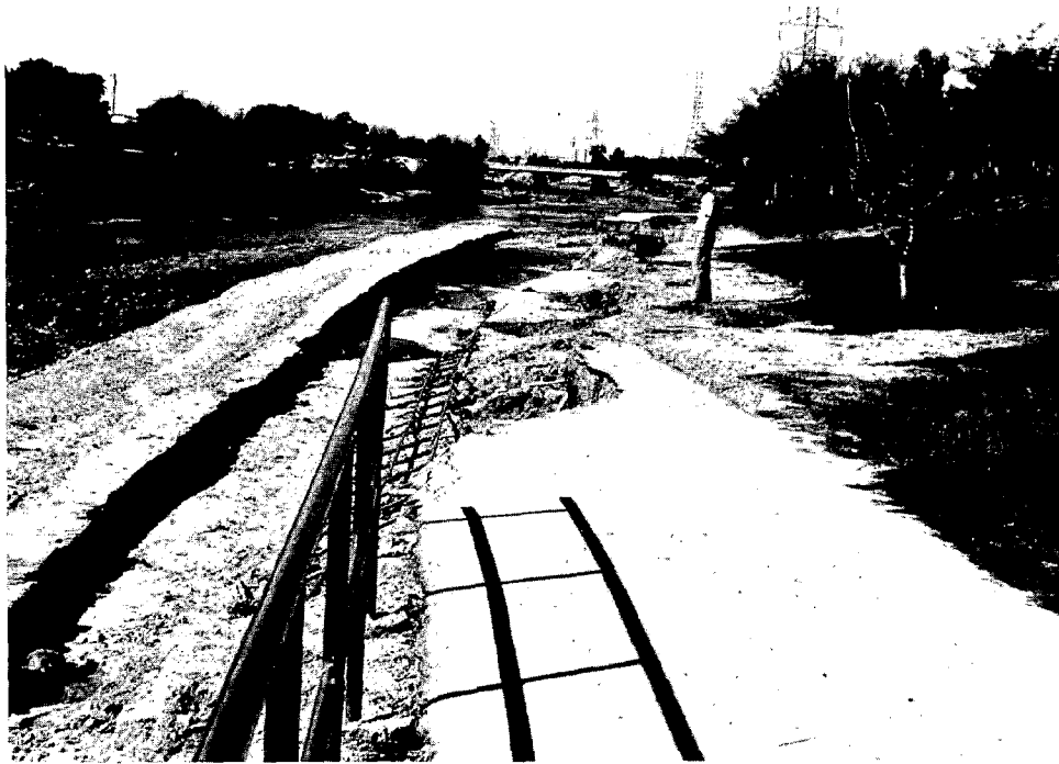
FIGURE 34 View downstream (north) along the Santa Cruz River between the St. Mary's Road bridge and the Speedway Boulevard bridge (visible at top center) on October 10, 1983. The distal terminus of the soil-cement bank protection has been eroded by the flows shown in Figure 33A. Photograph by Thomas F. Saarinen.
