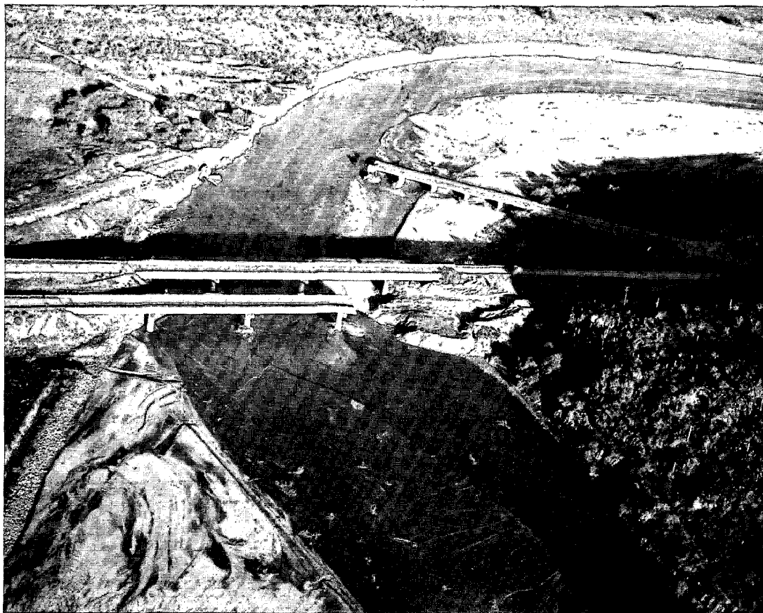
FIGURE 17 The Santa Cruz River at Martinez Hill (lower right) on October 9, 1983. Damage to the north abutment of the north-bound lane bridge of Interstate 19 is visible at center. As the flow meandered to the west bank, it eroded the west abutment of the San Xavier Road bridge (top center). Bank erosion extended through the former intersection of San Xavier Road and the access road to Interstate 19 at left center. Note the blocks of collapsed bank material on this bank. Riprap placed along this bank failed to prevent meander migration in the 1983 flood. Photograph by Peter Kresan.
