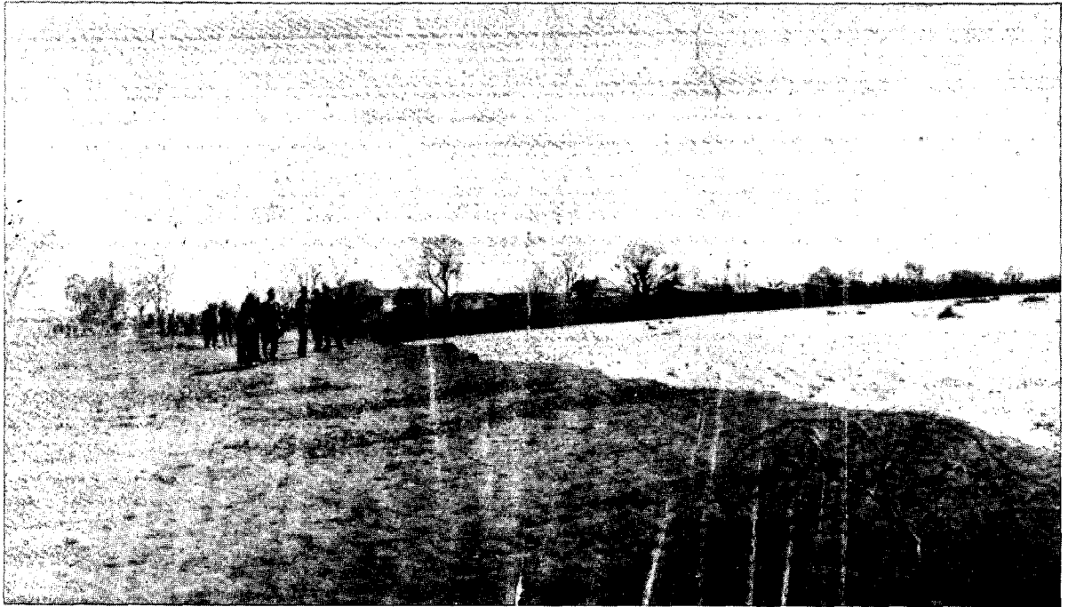
FIGURE 12 Erosion damage to the east abutment of the Congress Street bridge on February 1, 1915. The view is upstream (south), and Sentinel Peak ("A" Mountain) is visible at right. The gap of 60 m from the bridge to the east bank (left in picture) resulted from the downstream migration of a meander bend on that bank. This meander bend was visible in a 1902 photograph (Betancourt and Turner, in press). Source: Arizona Historical Society, Tucson.
