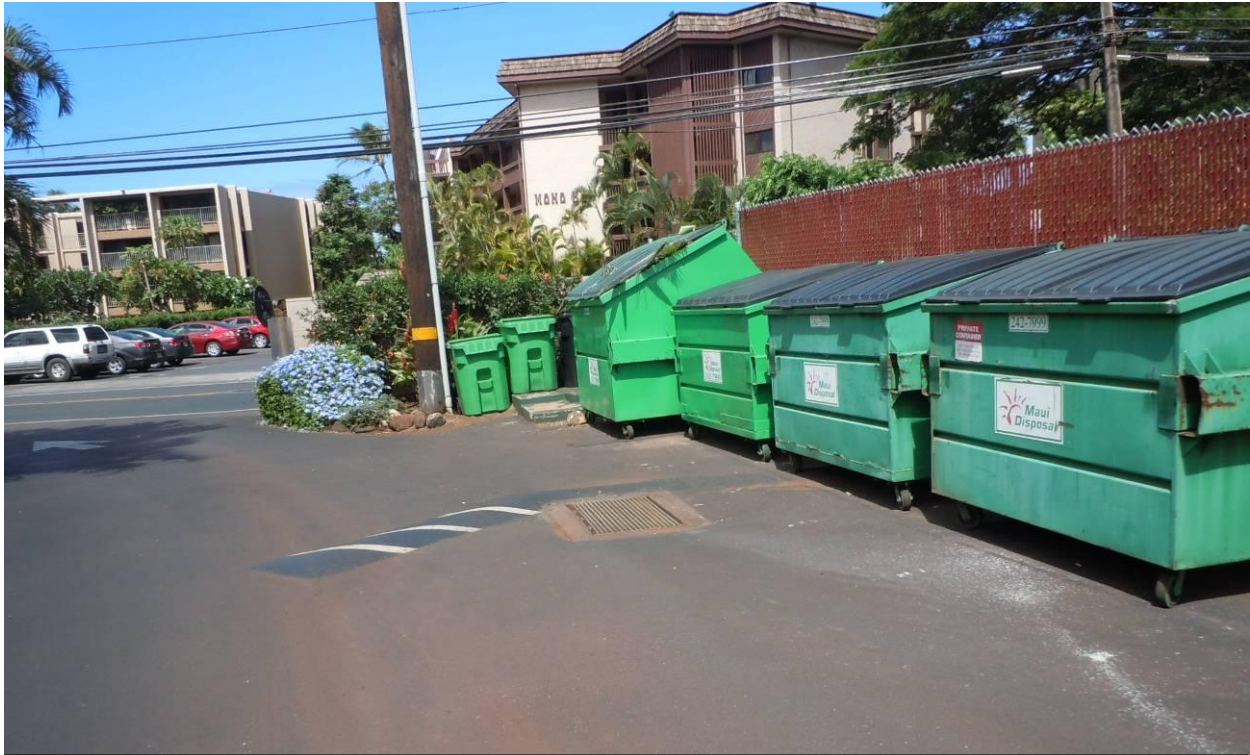
All of the dumpsters for this large complex (Hale Royale) are located right next to this catchbasin. The dumpsters do have lids, but there is still a risk of “dumpster juice” leaking directly into the storm drain.
