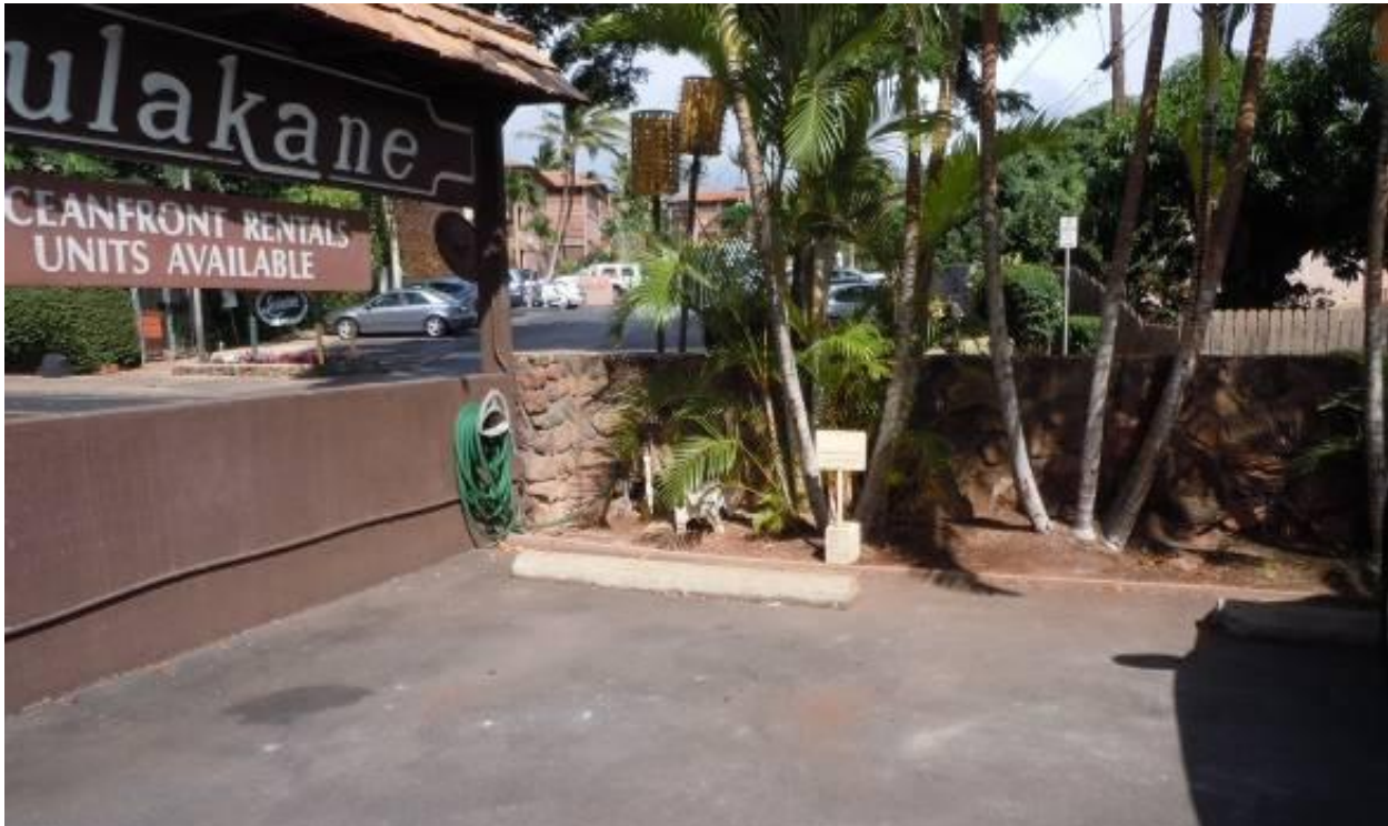
This is the identified (see sign) "Car Wash Station" at the Kulakane. Runoff from this area flows to the low point in the parking lot and out into Lower Honoapiilani Rd.
