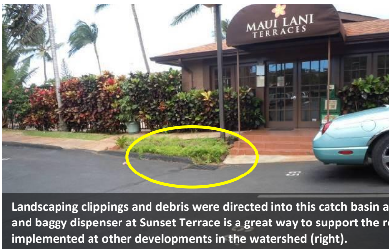
This catch basin is located in the landscaping area at Sunset Terrace near the back of the Farmer's Market Plaza. Flat grates like this one are easily clogged by vegetative debris, which can lead to flooding issues as well as adding more nutrients to the stormwater system.
