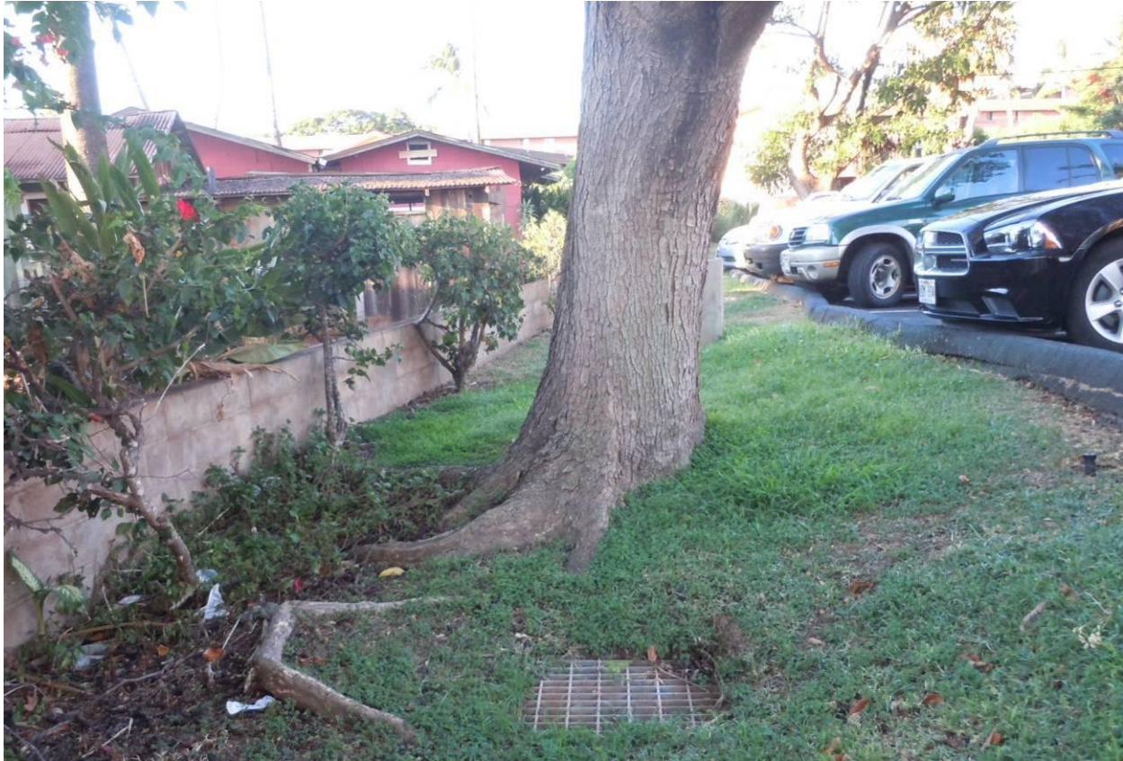
This catch basin is located in the landscaping area at Sunset Terrace near the back of the Farmer's Market Plaza. Flat grates like this one are easily clogged by vegetative debris, which can lead to flooding issues as well as adding more nutrients to the stormwater system.
