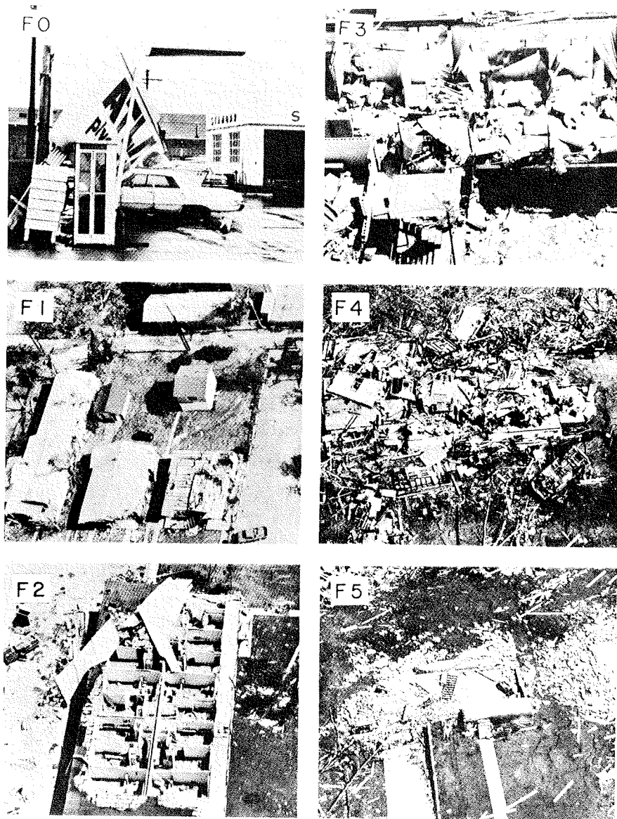
Figure 4.2 Damage intensity examples used for F-scale determination (from Fujita, 1978a).
