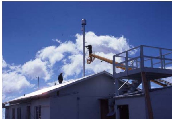
Putting up the new aerosol intake
