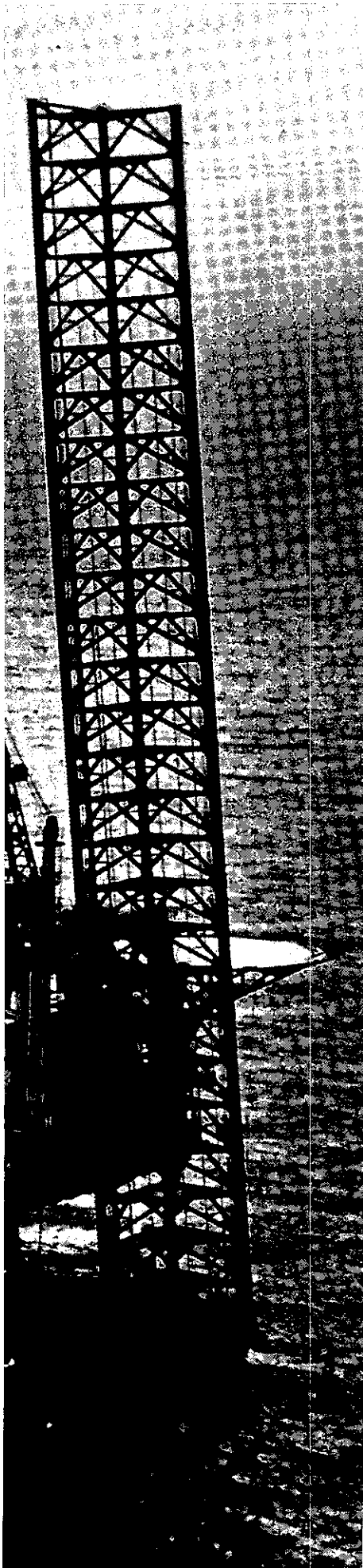
Left: Lowering the legs of a mobile oil exploration platform.
