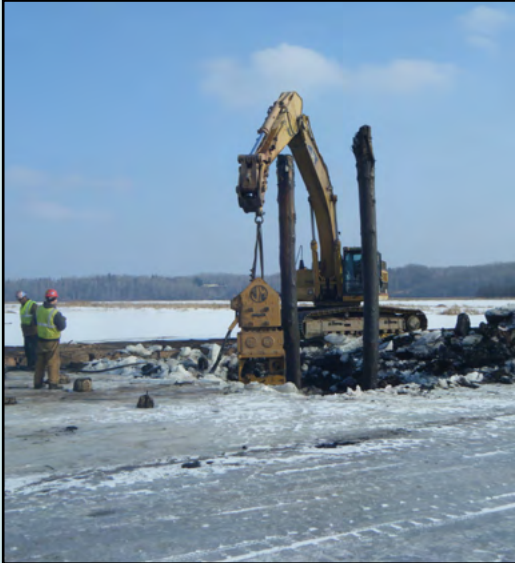
Heavy equipment removes debris from Radio Tower Bay.
