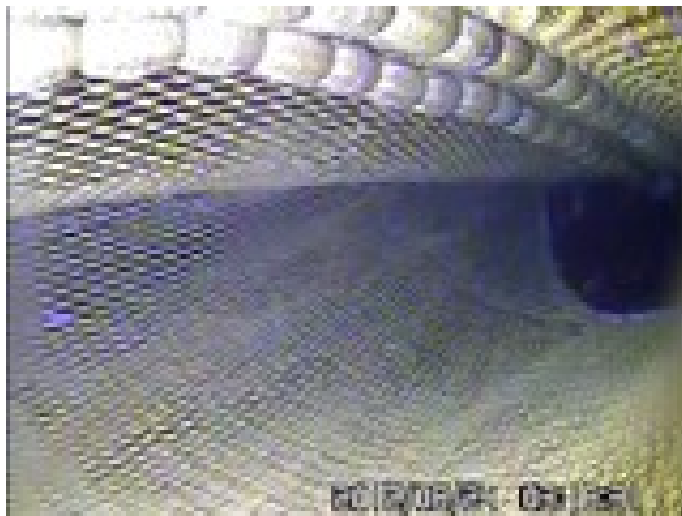
Figure 24. Lower escapement panel and scoop. Note float rope at the top of the figure.
