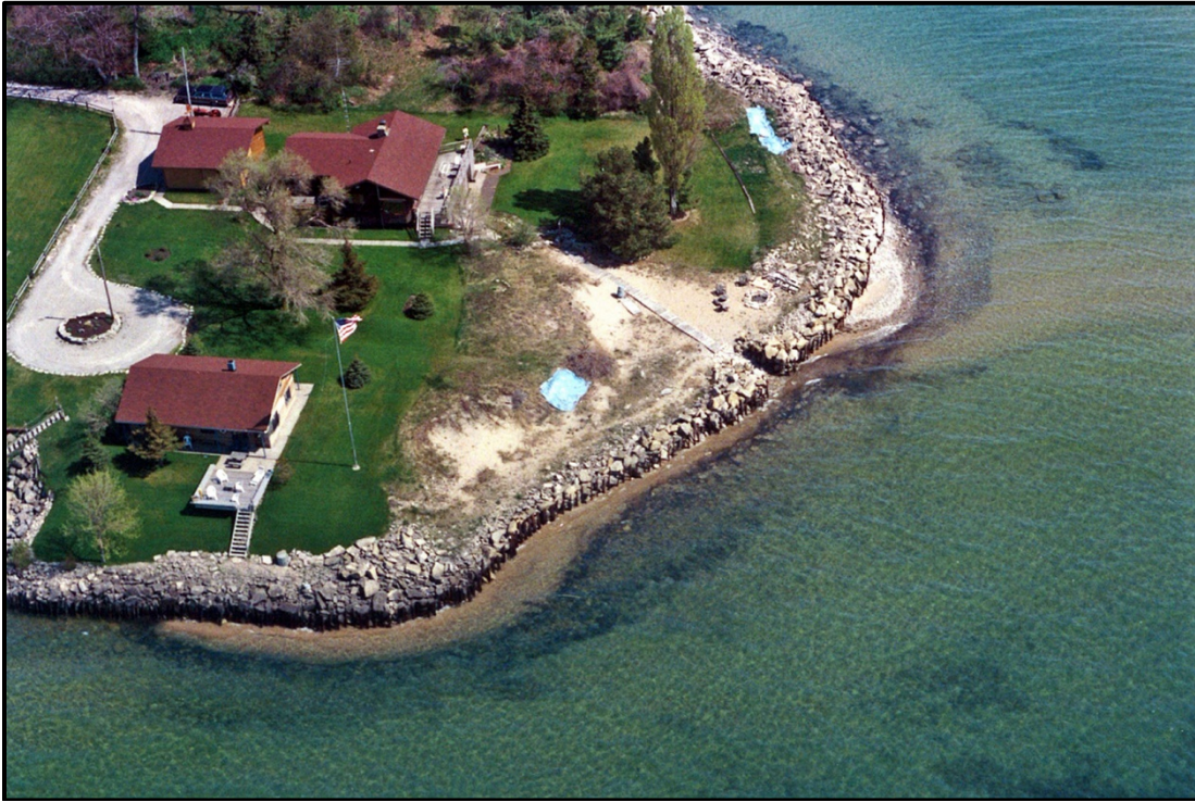
Figure 2.18: Riprap with ESI rank of 6B.
