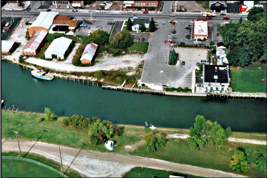
Figure 2.22: Sheltered, Solid Man-Made Structures with ESI rank of 8B.
