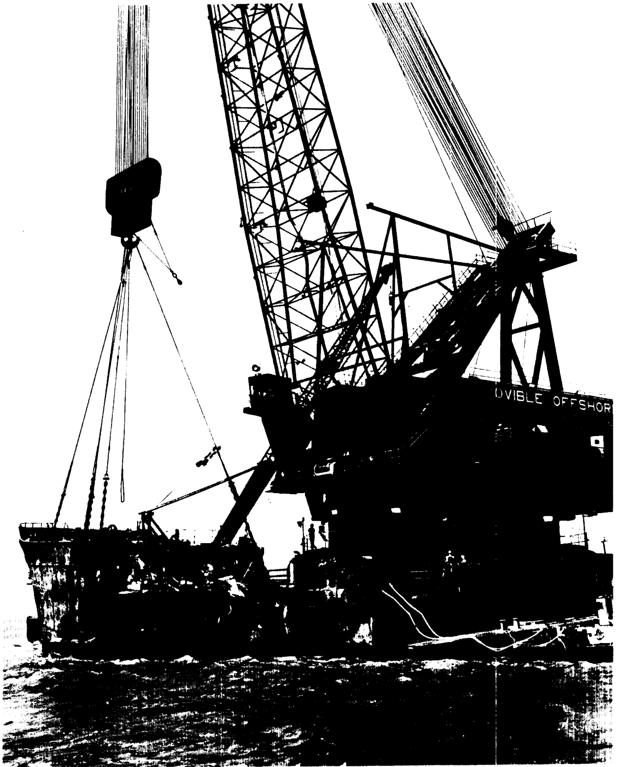
Fig. 11. Bow lift by 500-ton offshore crane.
