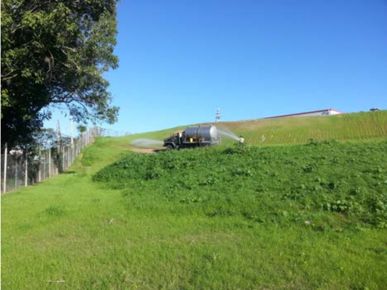
Figure 10. Vegetative stabilization and watering at the hardware store site
