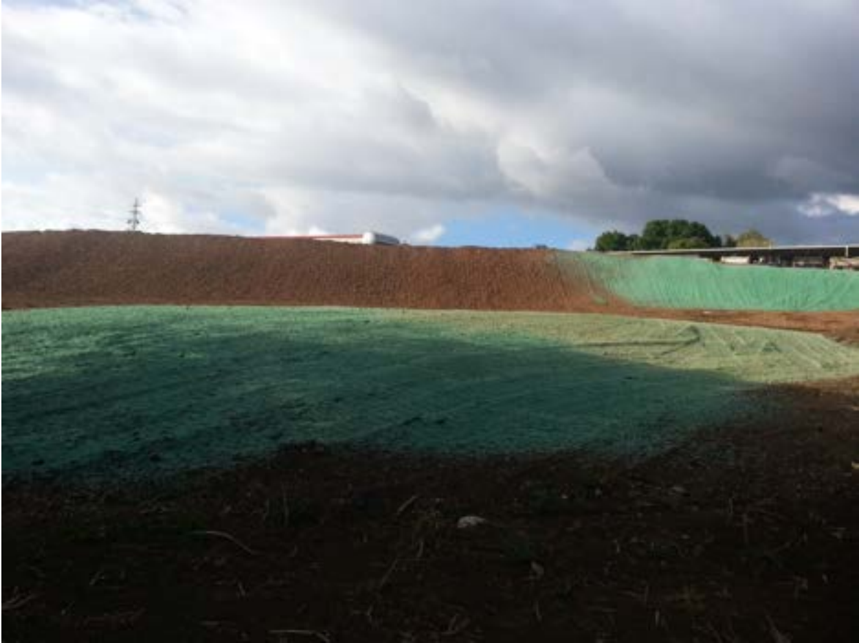
Figure 7. Hydroseeding in process at the hardware store site
