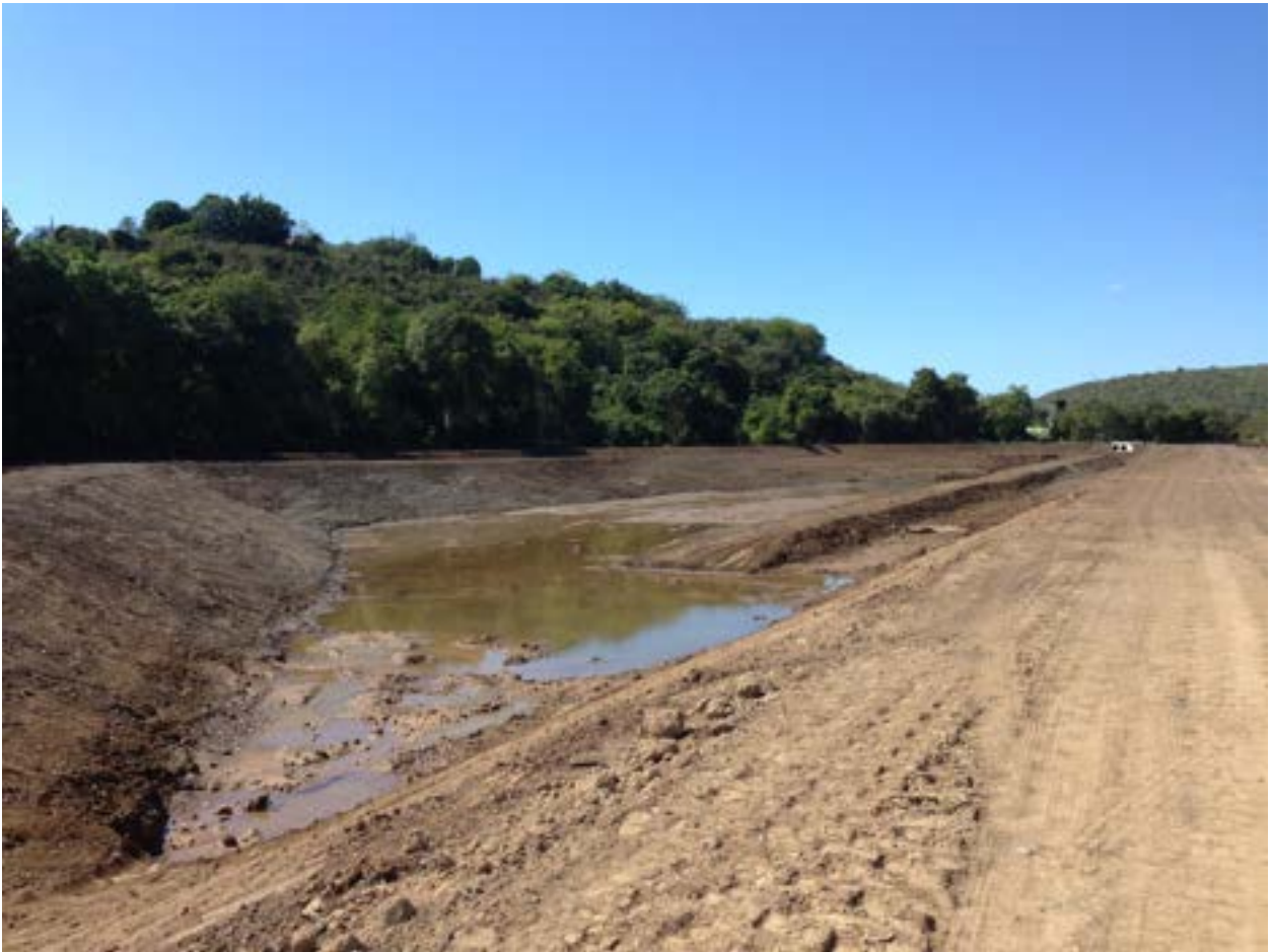
Figure 2. Sediment pond prior to stabilization efforts
