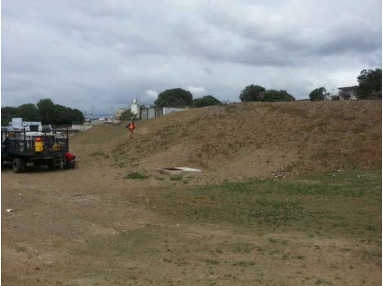
Figure 6. Preparing the site for hydroseeding
