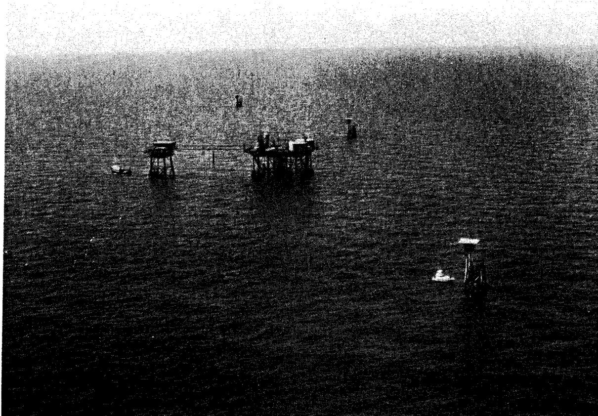
Fig. 2. A portion of the Buccaneer Gas and Oil Field showing the active 296 production platform and attached quarters platform, several satellite jacket wells and the small flare stack across from the catwalk.
