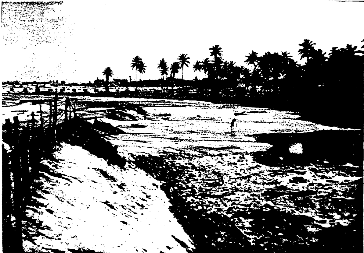
Figure 7-6B. View west toward Hatillo, transect V showing extensive washover zone, Oct. 13, 1982.
